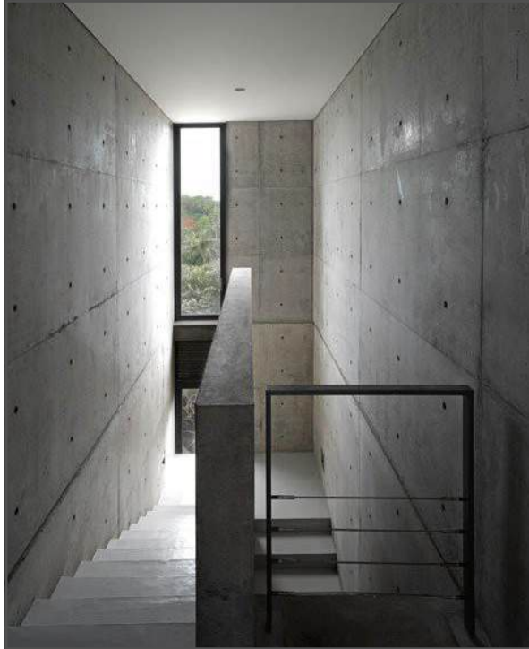
Fig. 8.3 Use of fair-face concrete in the interior
