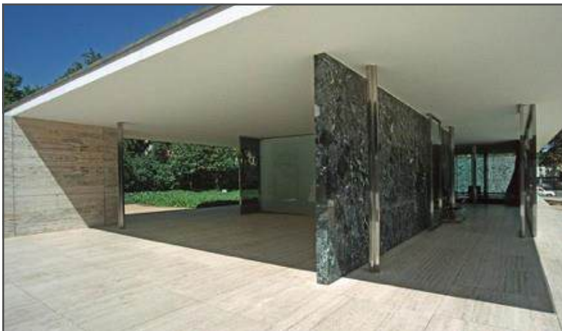
Fig. 2.4 The structure of Mies van der Rohe's Barcelona Pavilion rests on a plinth of travertine.
