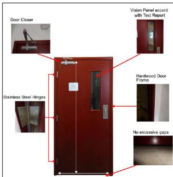
Fig. 3.11 A typical fire rated door. (Source: Buildings Department)
