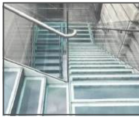
Fig. 4.8 This barrier-free handrail runs around the corner
