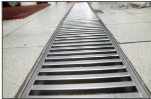
Fig. 7.3 Floor drain
