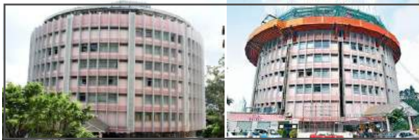
Fig. 2.11-13 Adventist Hospital mezzanine floor addition (Source: Adventist Hospital, Stubb's Road website)
