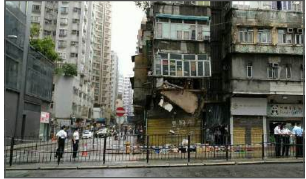
Fig. 2.1 Aftermath of a collapsed subdivided flat in Hung Hom in 2017 (Source: Ming Ming So via Facebook)
