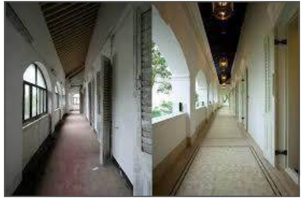
Fig. 9.7 Before and after revitalisation work on the corridor
