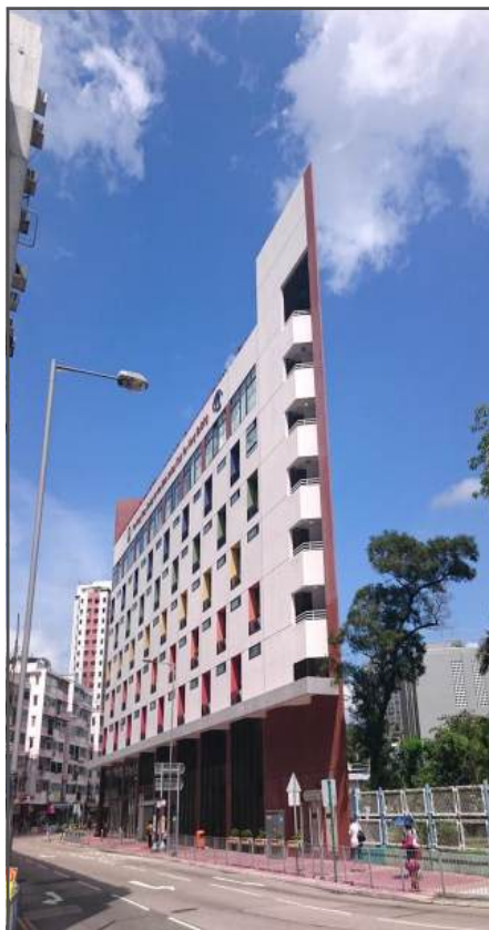
Fig. 8.2 Yuen Long Home for the Aged Blind
