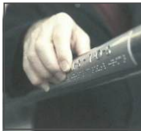
Fig. 4.10 Tactile information at the end of a handrail
