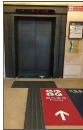
Fig. 4.26 Tactile Warning Strip to elevator
