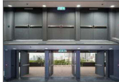
Fig.4.33 Emergency escape door
