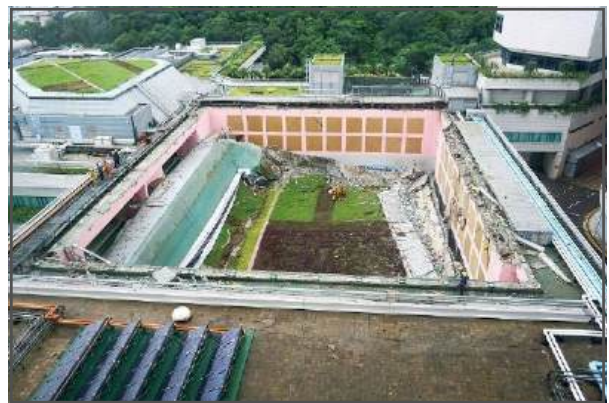
Fig. 3.1 Collapse of the roof of Hu Fa Kuang Sports Centre at City University in 2016
