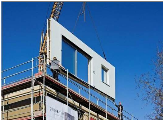
Fig. 5.1 Pre-fabricated housing materials
