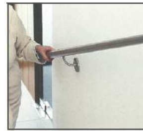
Fig. 4.11 Barrier-free, allround grip handrail
