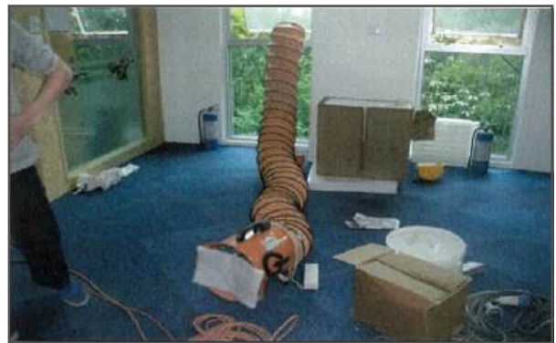
Fig. 5.4 Provision of fresh air during construction.
