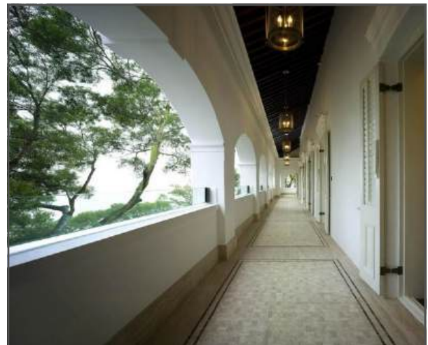
Fig. 9.4 Glass panels were installed on the railings along the corridor for extra height.
