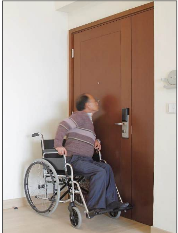
Fig.4.50 Peep-holes on doors are installed at both of the standing and wheelchair levels
