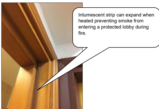
Fig. 3.12 Intumescent strip installed on a door frame of a smoke lobby door.
