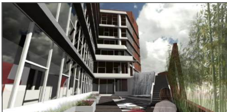
Fig. 8.6 Yuen Long Home for the Aged Blind (Jockey Club Yan Hong Building)
