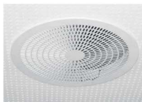
LPA Circular ceiling air diffuser for supply or extract air.
