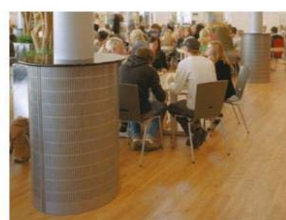
DCP Varizon® Displacement unit with adjustable diffusion pattern.
