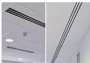
SWAN/SWAN WTW Rectangular linear air diffuser for supply and extract air.
