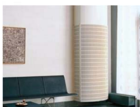
DBC Varizon® Displacement unit with adjustable diffusion pattern.
